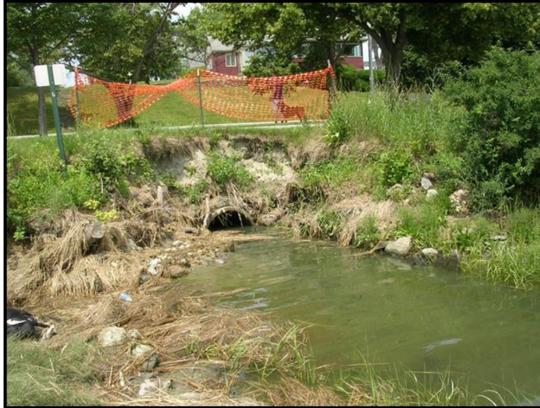
CSO 10, Mackworth Street Discharge to Back Cove Replaced in 2009
