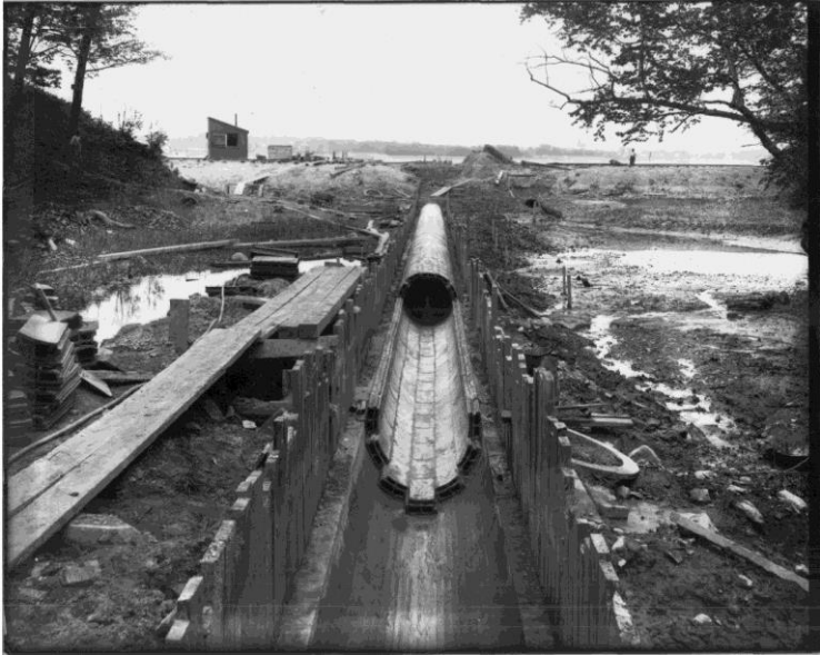
Portland, Dartmouth Street Combined Sewer, 1918
