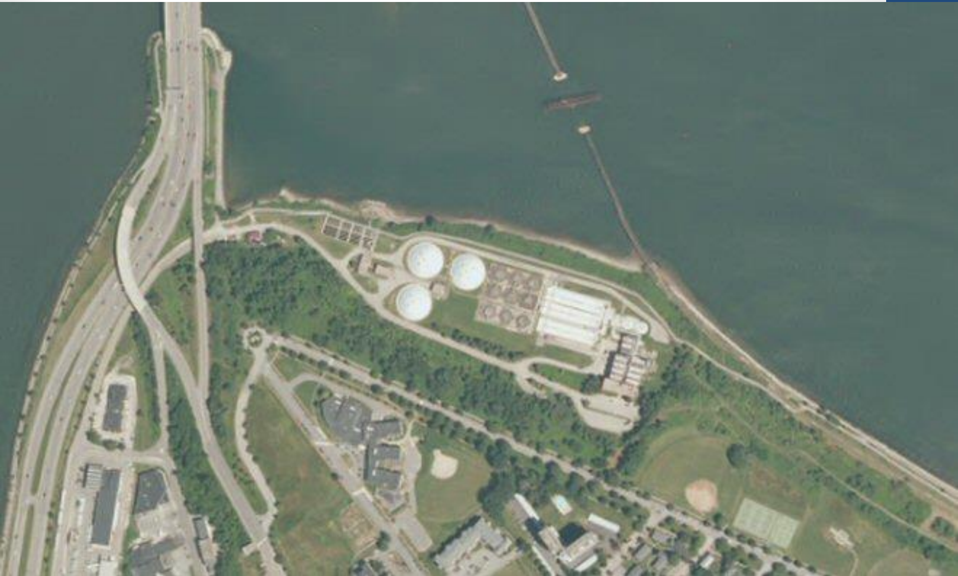
East End Treatment Plant – est. 1979
